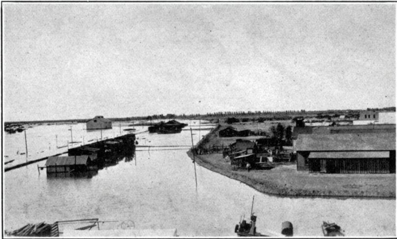
Flood scene showing the levee.
